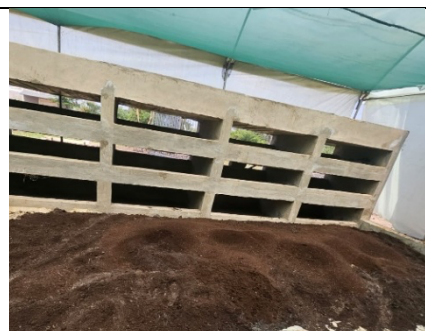
Figure 4. Concrete trays were built by local farmers
