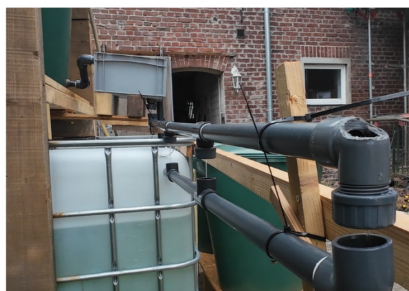
Figure 3: The supply line to the cultivation systems must be designed with a slight slope to ensure sufficient flow. This allows the individual outlets to fill with water and the excess water to flow quickly to the next outlet.
