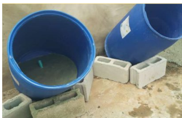
Figure 2: Filter seen from inside
