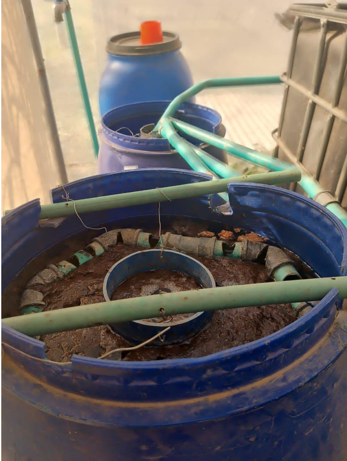
Plate 3.3 Radial flow tank
